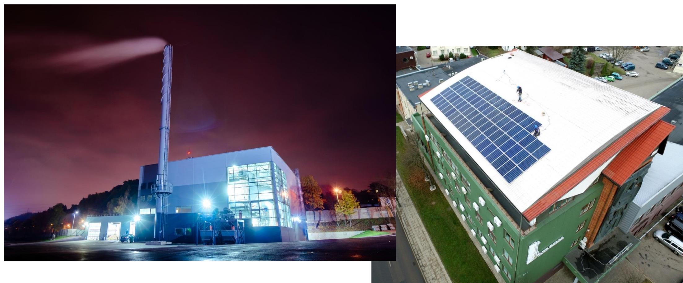
Figure 1. Biomass boiler-house of independent producer and Solar PV on the roof of AB Kauno energija
